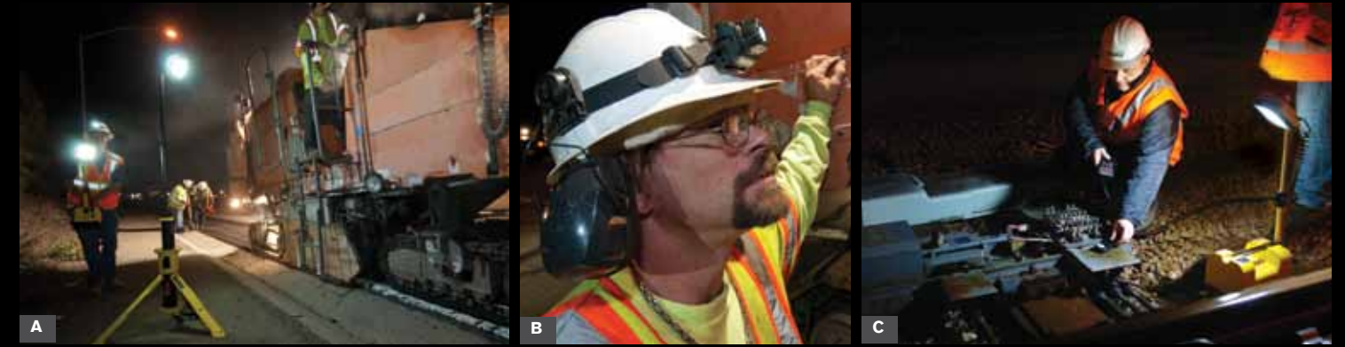
Photography: Caltrans Highway Repair Crew (A, B), Rail Worker (C).
